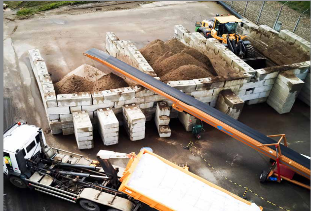
Sorting potentially contaminated soil
