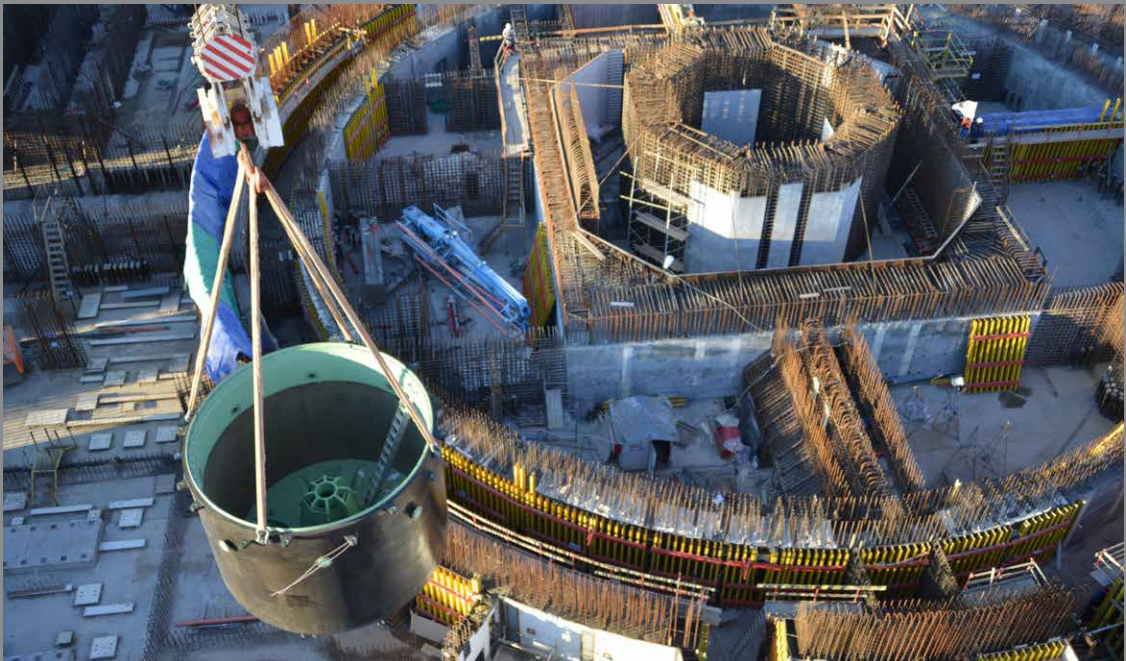
Installation of a Melt Trap at the Kursk Npp-2 Under Construction
