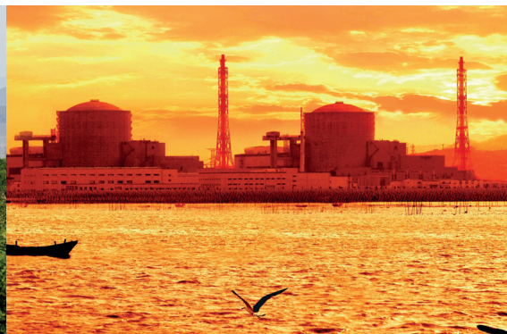
TIANWAN NPP (CHINA)
